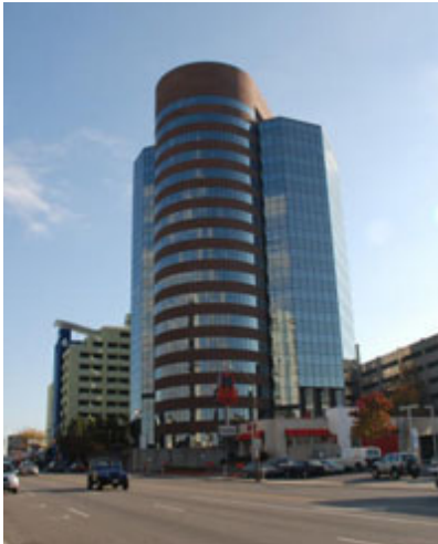
Palmer Plaza Building view from West End
